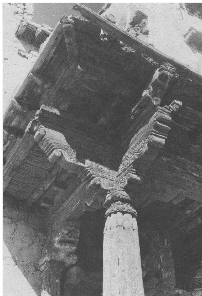
FIGURE 7. The main entrance porch on the eastern side showing the unusual canopy and elaborately carved timber; probably of Kashmiri influence, it depicts the Snow Lion which was the emblem of the builder.
